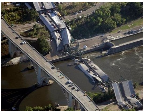
Figure 3 The Minnesota I-35W highway bridge collapsed on August 1, 2007 (photo credit unknown). The NTSB Go Team was headed by Investigator-in-Charge (IIC) Mark Bagnard. Mark Rosenker, Chairman at the time, was the spokesperson accompanying the Go Team on the scene. Source: NTSB Annual Report (2008, page 54). See Appendix A.6 for details on the accident and investigation.
